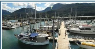
Aurora Harbor Rebuild, Juneau
