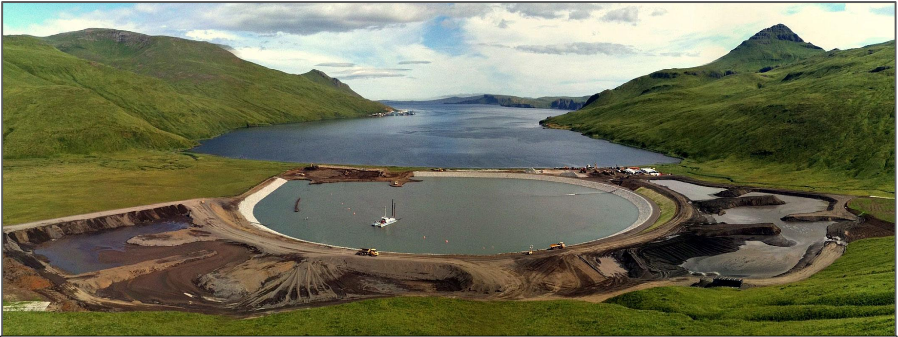
USACE Alaska District constructed a harbor at Akutan in the Aleutian Islands between May 2011 and October 2012. The $31.9 million project established an entrance channel and mooring basin, along with two rock breakwaters. USACE ALASKA DISTRICT PHOTOS
